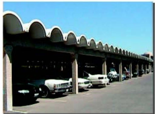
FRP Roof for Car Parking
