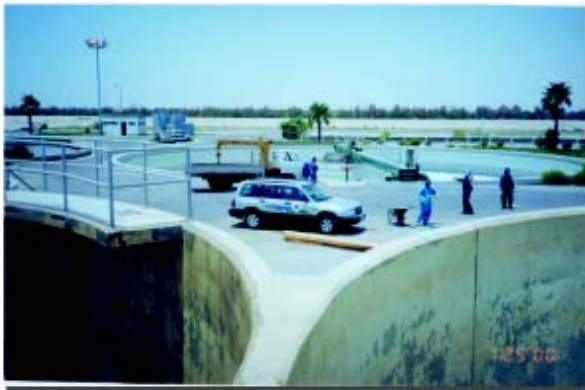
FRP Coating for Sewerage Treatment Tank
