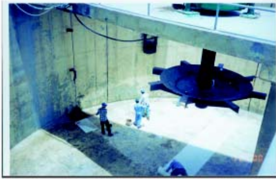
FRP Coating for Sewerage Treatment Tank
